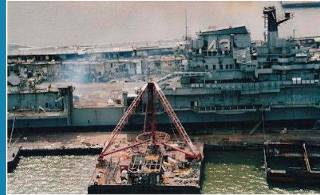
PIER BREAKING / ALONGSIDE
